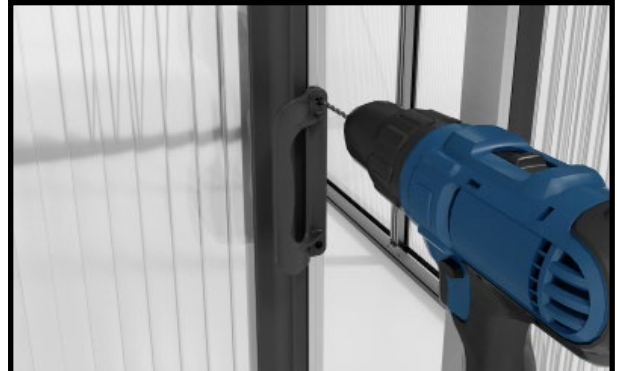
Start with the outer door handles. Pre-drill holes with a 4 mm drill bit.
