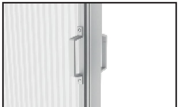
The installation of the door is completed after fixing the door handles inside and outside.
