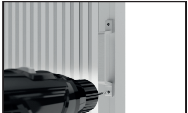
Pre-drill holes with a 4 mm drill bit.
