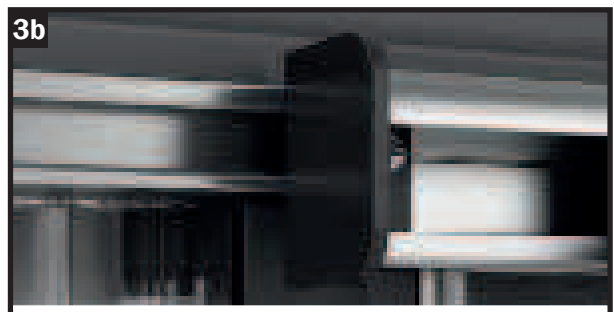
Fix the door rail guard onto the door rail. Screw the door rail with the drilling screw so that the door rail guard is firmly held in the door rail. Place the drilling screw in the V-groove of the door rail.
